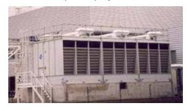
Typical induced draft, cross-flow cooling tower.
